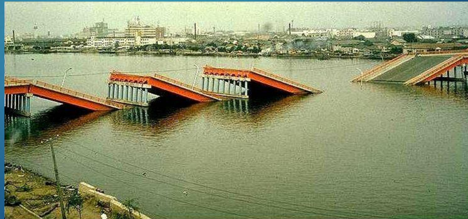
1964 Niigata, Japan Earthquake
